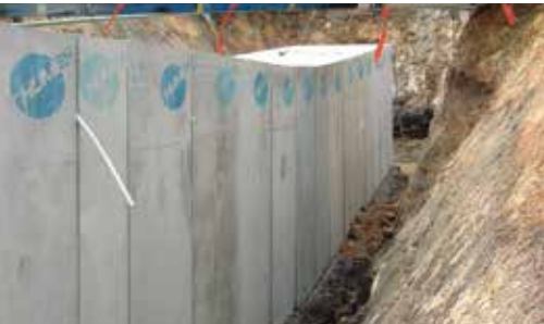
Manukau Police Hub Tunnel, Manukau City, New Zealand
