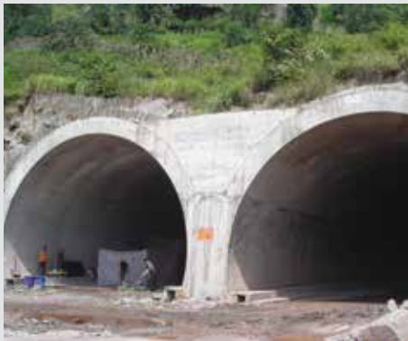
Repair work on the Yunnan Shuima Tunnels
