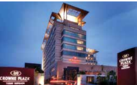
Crowne Plaza Hotel, Below grade & swimming pool, Gurgaon, Haryana, India
