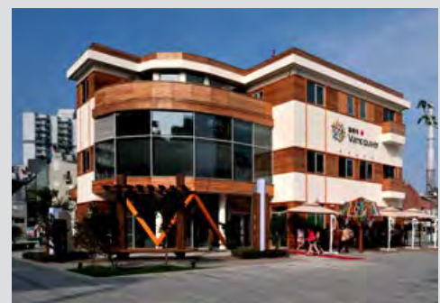
Vancouver Pavilion, Shanghai, China
