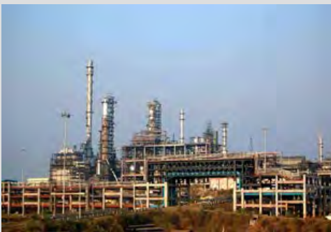
Bharat Oman Refinery, Bina, India
