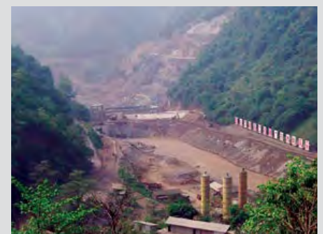
Madushan Dam, Yunnan Province, China
