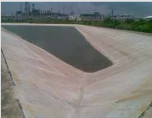
Repair work on the Bharat Oman Refineries, Bina, Madhya Pradesh, India
