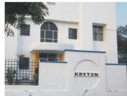
Kryton-India factory, Dharuhera, Haryana.
